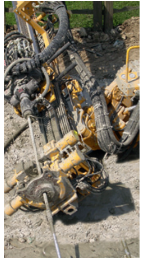
Rotary percussive drilling for DYWI® Drill soil nails
