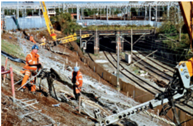
Long reach excavators with hydraulic powered drill booms for soil nailing
