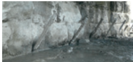
Raking micropiles for bridge pier upgrades
