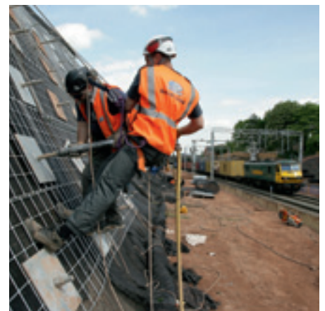
Plating up, using pneumatic box wrench
