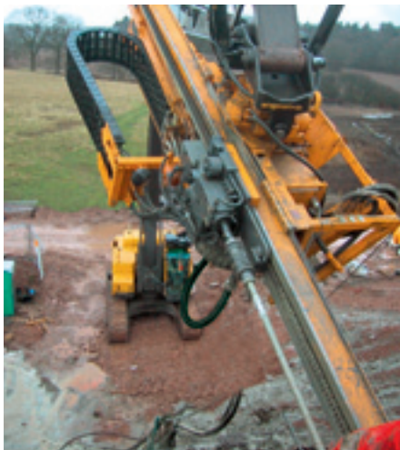
Drilling with long reach excavator
