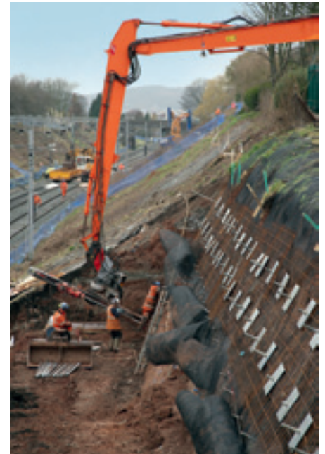
Long reach excavator for restricted access drilling
