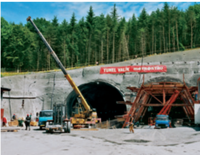
Installation of 67,000m of DYWI® Drill Hollow Bar Anchors, Ø 25mm – Valik Tunnel near Pilsen, Czech Republic
