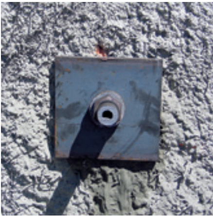
Stabilization of a trough structure using DYWI® Drill Hollow Bar Anchors, Ø 38mm – Reno, Nevada, USA
