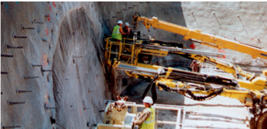
Self-drilled hollow bars for the stabilization of a tunnel portal and approach cutting
