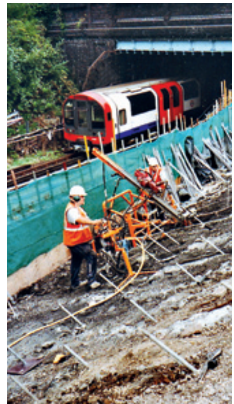
Restricted access soil nailing
