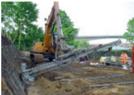
Excavator mounted drill boom, installing top bar galvanized soil nails
