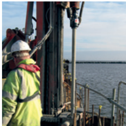
Grout injection behind sheet piles
