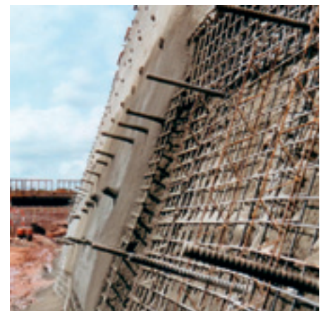
Grouted soil nails on shotcrete face
