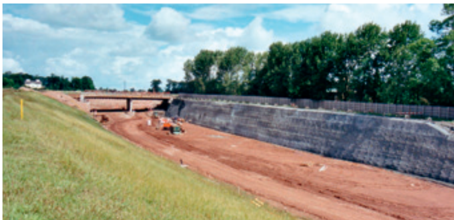
Steep cut slope with shotcrete facing for structural stiffness to resist bulging
