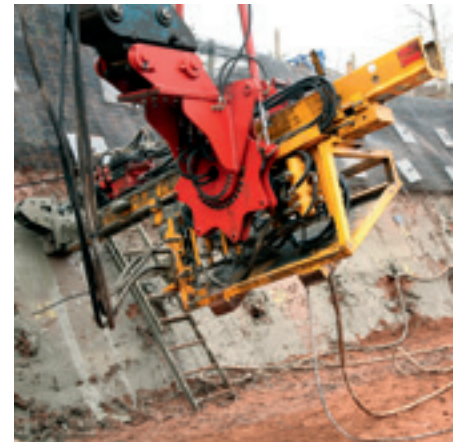
Excavator mounted drill boom for versatile positioning of the soil nail
