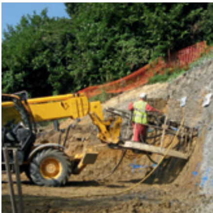
Drill platform mounted on telescopic forklift
