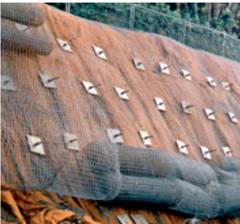
Hollow bar rock bolts for stabilization of a weathered face
