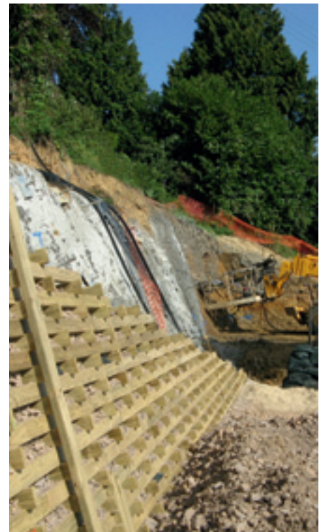
Soil nailed slope with crib wall facing
