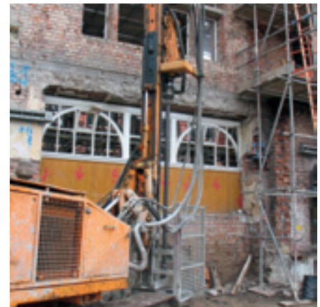
Micropiles for retained facade frame bases
