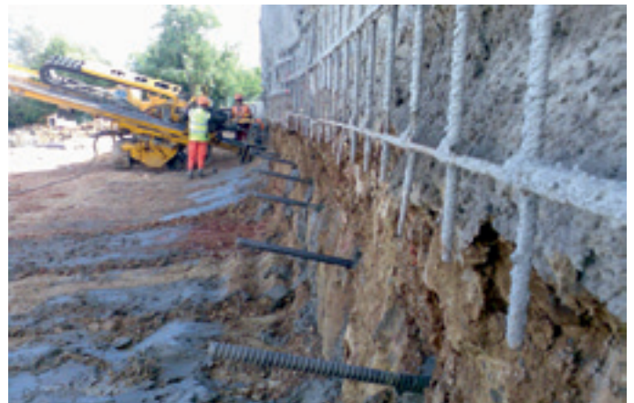
Top down construction using hollow bar soil nails and shotcrete
