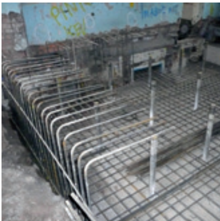
Base slab reinforcement using micropiles
