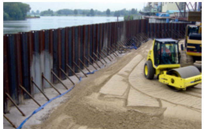
Sheet pile tiebacks using large diameter hollow bars
