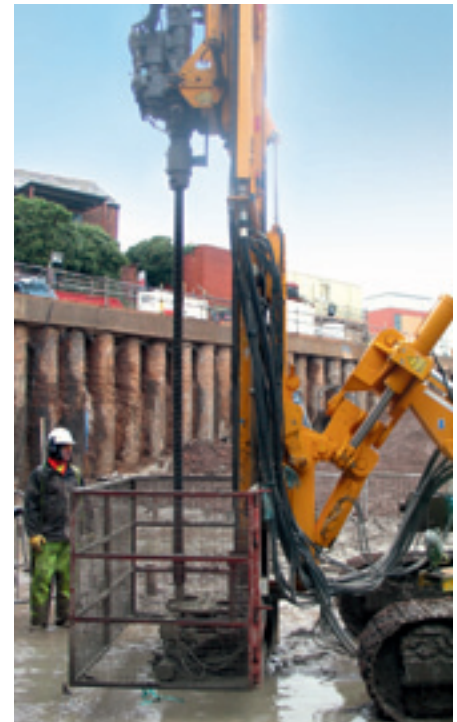
Long stroke drill boom for deep micropiles
