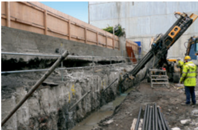
Drilling through a secant piled wall
