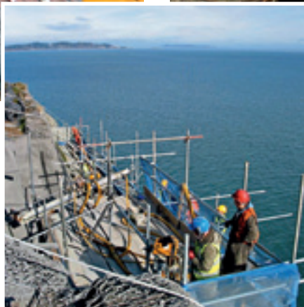
Scaffold mounted hydraulic drill boom for rock bolting
