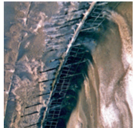
Hollow bar spiles installed through a lattice girder
