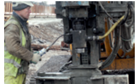
Greasing of seal tracks (H64/R51 adaptor)
