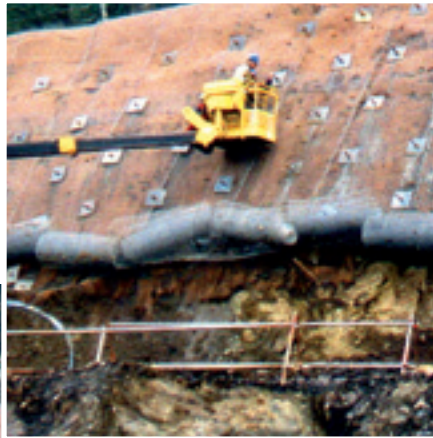
DYWI® Drill rock bolts for anchoring of rock fall netting
