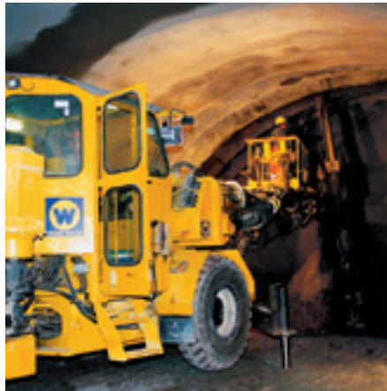
Stabilization of a tunnel portal using DYWI® Drill Hollow Bar Anchors, Ø32mm – Thuringia, Germany
