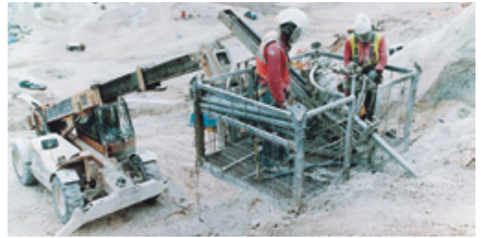
Installation of DYWI® Drill Hollow Bar Anchors at the Garden of Eden project in Great Britain
